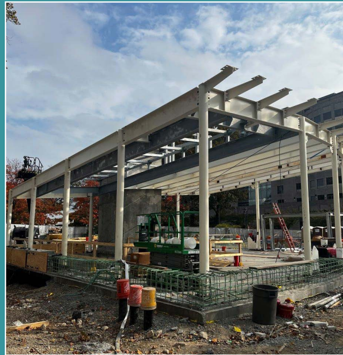
Structural steel for the headhouse is now substantially installed.
