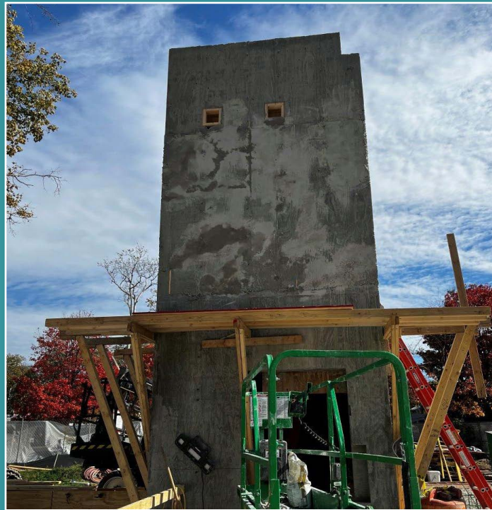
Concrete has been placed for the last segment of the elevator shaft.
